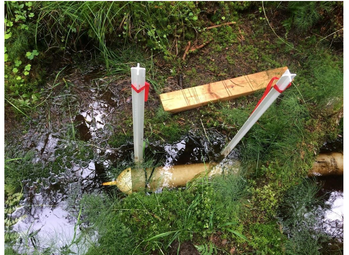
TIMS installed in an uncleaned ditch
